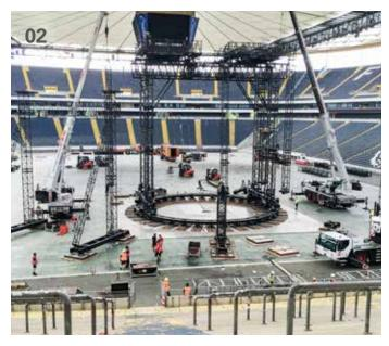
01 Multi-directional locking mechanisms allow for weight dispersal and minimize the risk of damage to and compaction of the subsurface | 02 Quick to deploy, the system provides high levels of protection for sensitive surfaces | 03 This drivable event flooring has a sandblasted, non-slip surface with a flat profile and is available in grey or green | 04 ArmorDeck 3 is suitable for indoor and outdoor use
