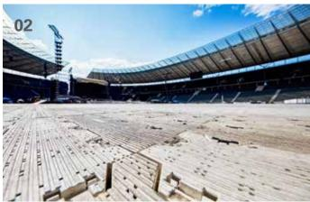
01 Supa-Trac is supplied in pre-fabricated layers of 15 which facilitates rapid installation | 02 The turf protection system is ideally suited for open-air concerts, stadiums or other large events with high spectator numbers | 03 Depending on weather conditions, Supa-Trac can protect turf from external influences for up to five days | 04 Supa-Trac's surface is permeable by light, water and air
