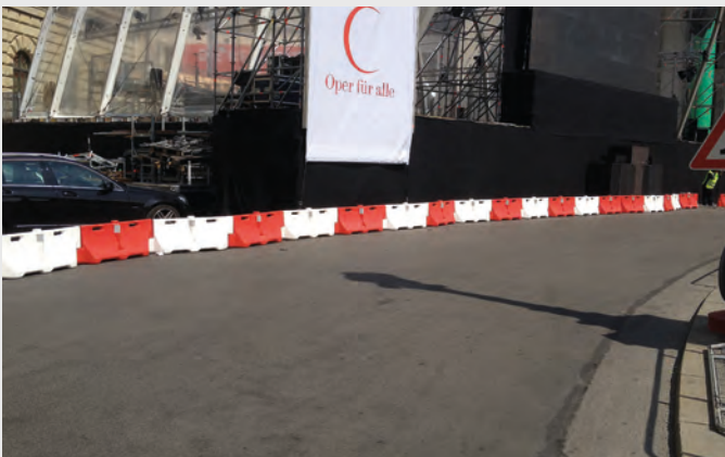
Temporary changes to the road system
