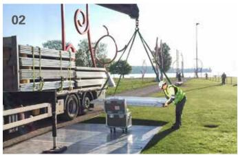
01 Box Panels withstand the heaviest loads | 02 The heavy-duty aluminium panels are laid and bolted together using a rear-loading crane from a crane truck | 03 Underlaid with special mats, Box Panels also provide protection for sensitive surfaces such as natural flooring | 04 Ramps ensure trip-free, smooth transitions
