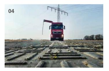
01 PistEco transforms yielding subsoils such as meadows and farmland into heavy-duty roads, access roads and assembly platforms that can be driven on by heavy trucks or construction machinery | 02 PistEco plastic panels adapt optimally even to soft subsoil | 03 In addition, the connected panels remain movable in relation to each other | 04 The panels provide both site access and an assembly platform simultaneously
