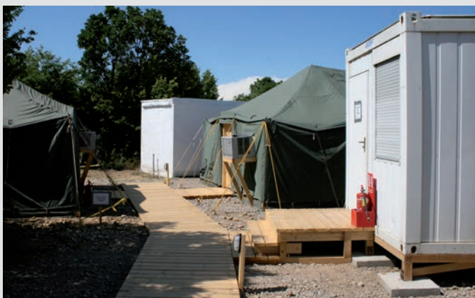
Temporary offices for a construction site
