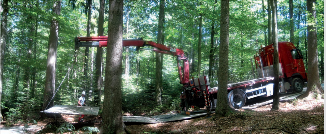
A HD panel access road running through a nature preserve
