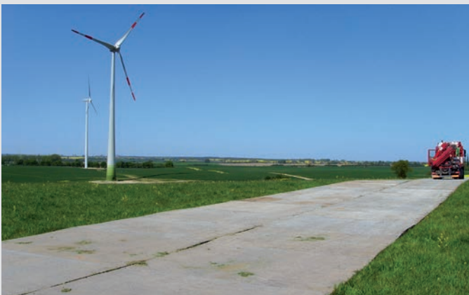
A HD panel access road for wind turbine installation
