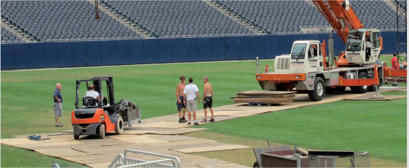
Temporary access road for forklifts and cranes
