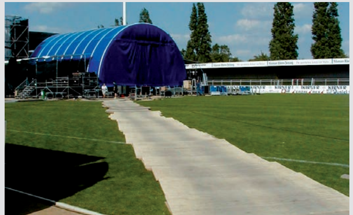
A plywood transport path for rolling cases and supply vehicles
