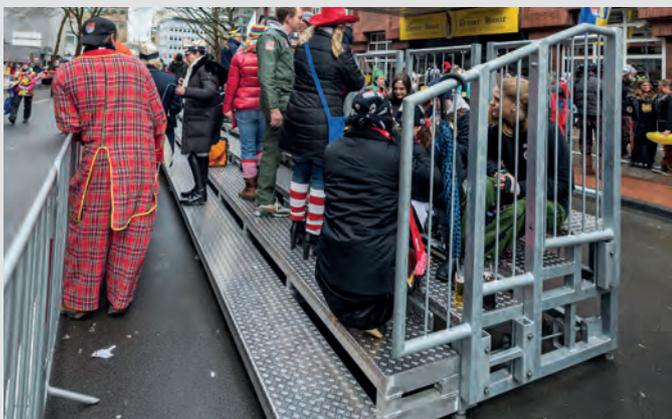
Only five steps are necessary to build the grandstand: unloading, positioning, connecting, unfolding and mounting the handrail
