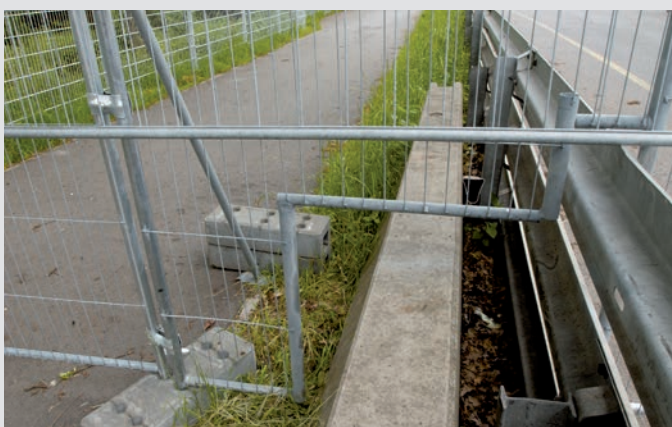
A custom-made fencing element at FIFA WM 2006
