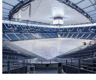
01 With semi-automated laying machines, Arena Light Panels can be installed extremely quickly, safely, costeffectively, and sustainably | 02 Simply lift, place, screw, done | 03 The pedestrian-friendly heavy-duty plates can cover entire stadium fields, as seen here at the Deutsche Bank Park in Frankfurt am Main | 04 Stable connections and recessed screws create surfaces without any tripping hazards
